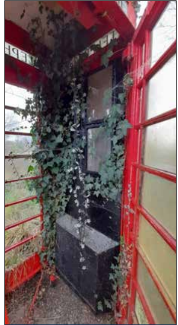
Before the renovation, inside the phone box
