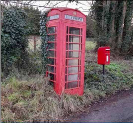
Before the renovation
